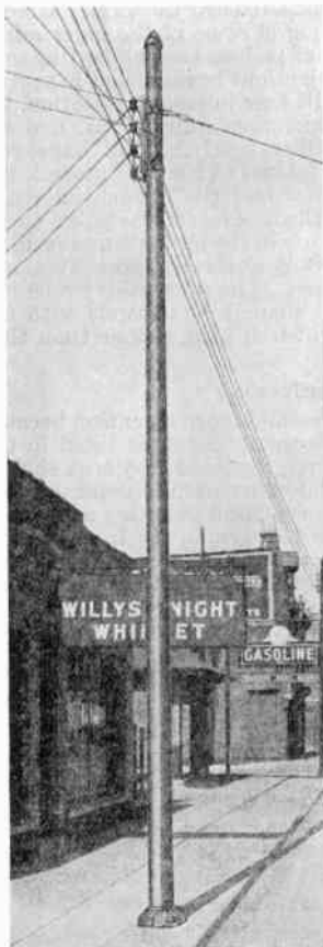
Semi-Ornamental Steel Base
