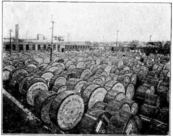
Cable Yard at Hawthorne Works
