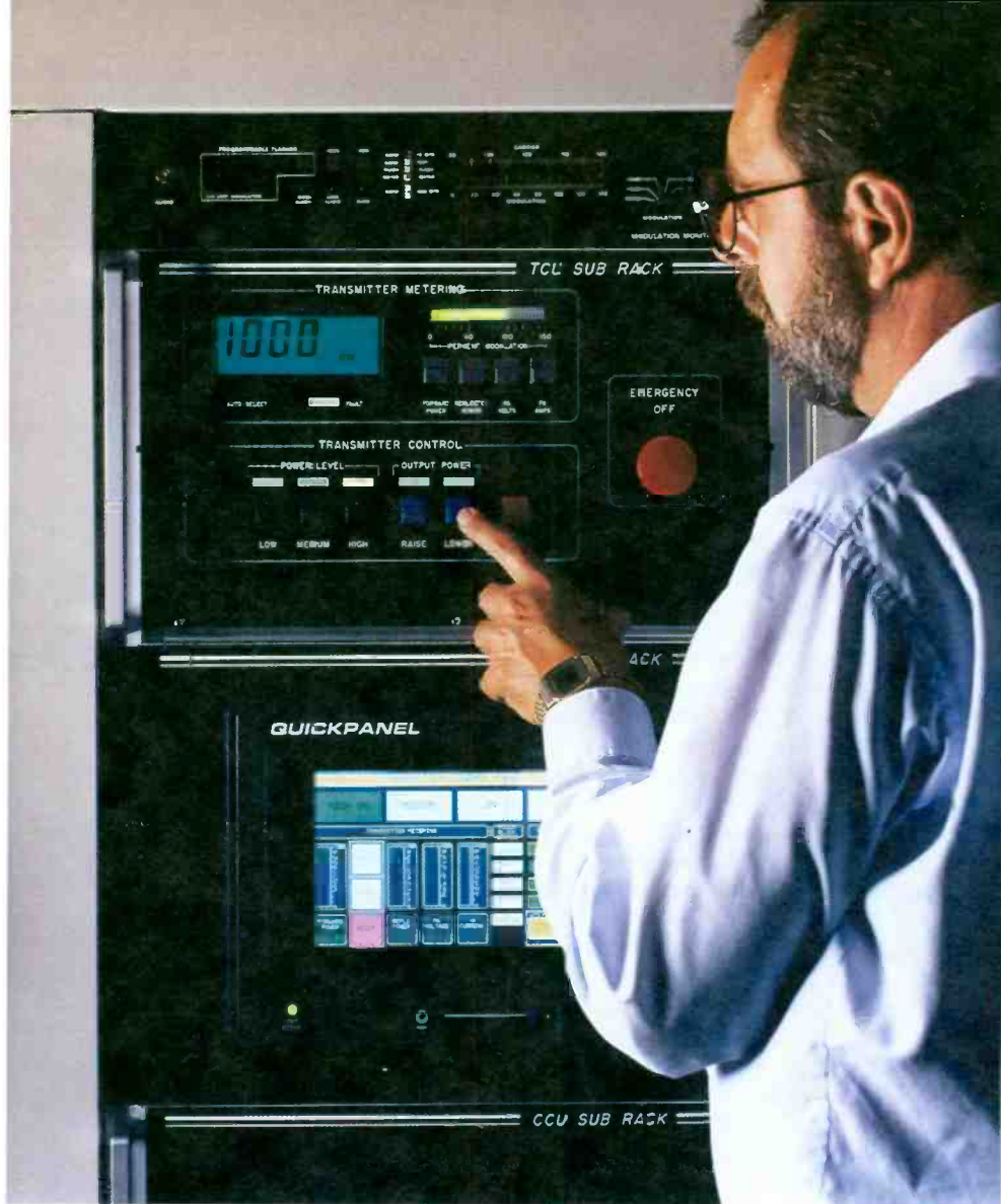
Digital Amplitude Modulation has made it practical to provide super-power solid state medium wave transmitters.
