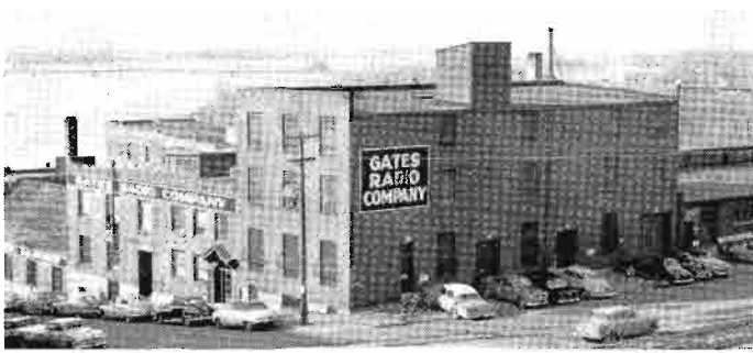
Gates Hampshire Street plant in Quincy, Illinois with 50,000 sq. ft. of manufacturing and administrative office space.
