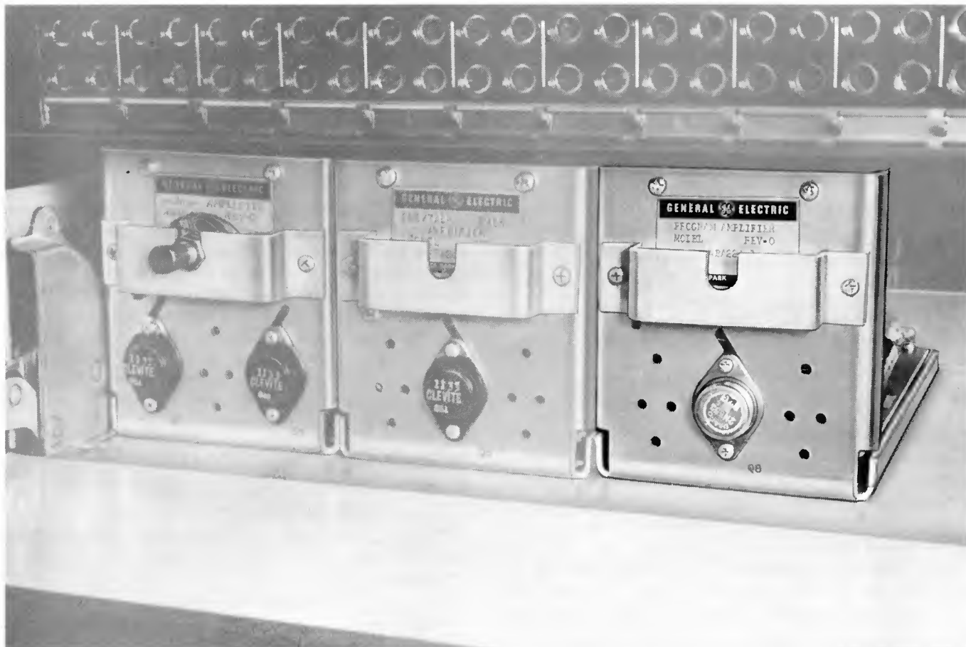
Type BA-22-A Program Amplifier installed in a Type FA-48-A Equipment Shelf.
