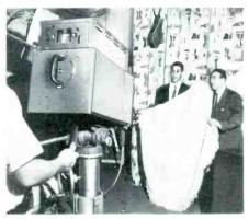
Program in progress. Vitaecan mobile camera is used in exactly the same manner as an ordinary camera. Operator focuses and views through electronic viewfinder.
