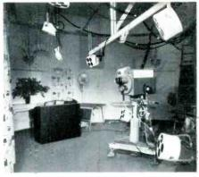
Typical studio scene ready for programming. No:e positioning of pickup scoops arranged to achieve back-lighting, highlighting and other dramatic effects.
