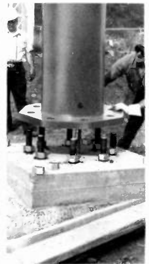
Pole in position to be lowered on plumbing nuts.
