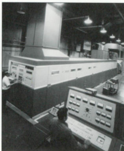
Top: FEBC Saipan 2 ea. 100 kW SW transmitters.
