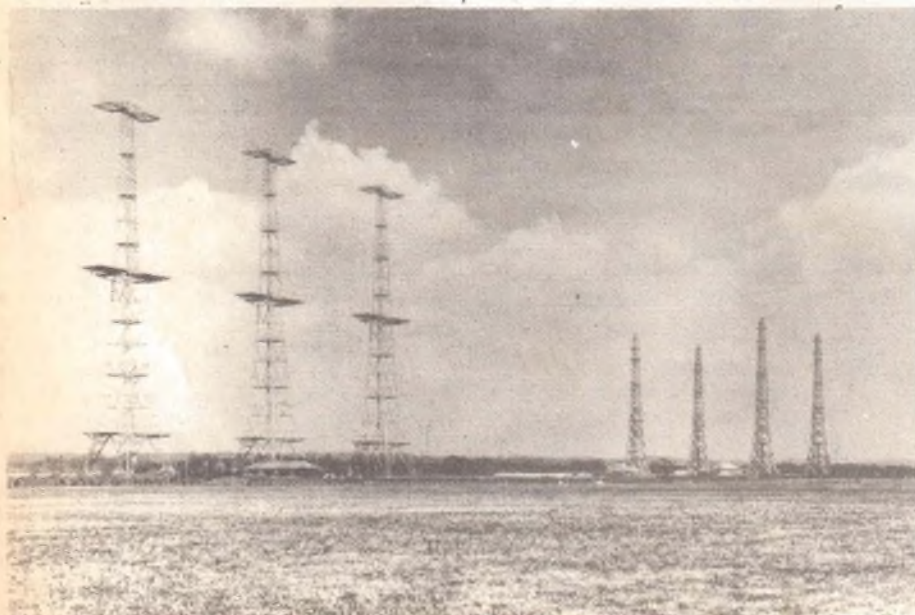
Fig. 3. Typical aerial system of operational coastal CH radio location station. The three large 350ft. high steel towers carry the transmitting aerials. The
