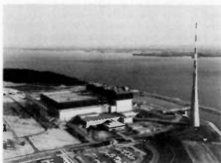
Large nuclear power generating facilities ("nukes") are getting to be familiar sights. This one, the Brown's Ferry facility operated by the Tennessee Valley Authority in Alabama, runs communications on a number of frequencies and lots of people wish you wouldn't listen in on them! Doesn't that make you curious?
