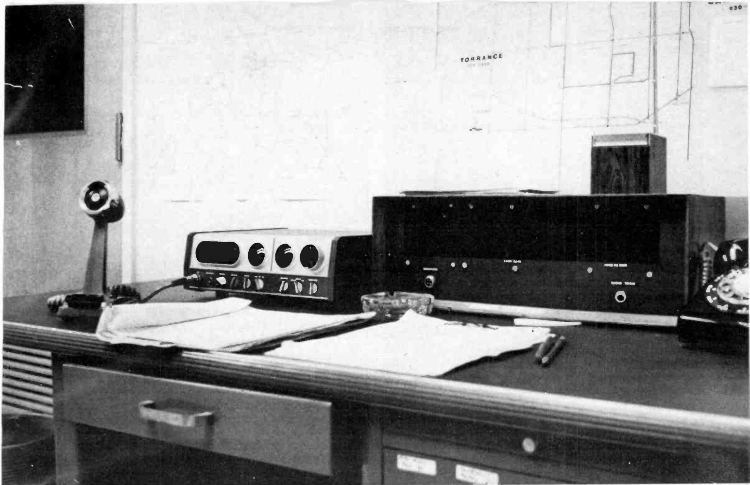
Here is the dispatch console for a program called "Neighborhood Watch," established by the police in Gardena, Calif. Such programs, while useful, must be operated at the discretion and under the direction of police authorities so they do not take upon themselves a distasteful "vigilante" flavor.
