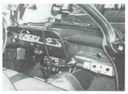
The mobile unit of Bob Bridges, KCG2486, of the Tri-County REACT Team. The unit is equipped with a 23 channel rig, a PA system, a sound system, police and fire call monitors, 117 VAC power supply—all neatly mounted below the dash.
