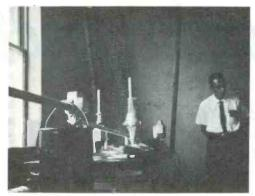
Snapped while nobody was looking. This is one of the torture tests, it consisted of a 69 lb. bucket of nuts and bolts which was hung on a horizontally mounted C-225 rotor. As it was maved further and further out on the pole, the effective weight load increased. It could go almost to 900 lbs., but they couldn't get the rotor to break.
