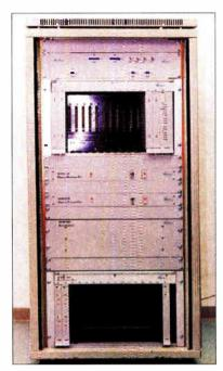
In the headend, GADline features a management interface unit, frequency transvertor and convertor units, a splitter combiner and a trunk interface unit.
