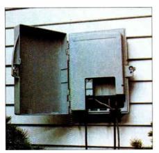
From the factory, ADC's basic Home Integrated Services Unit features one or two POTS lines (expandable to four) and provides for on/off video control.
