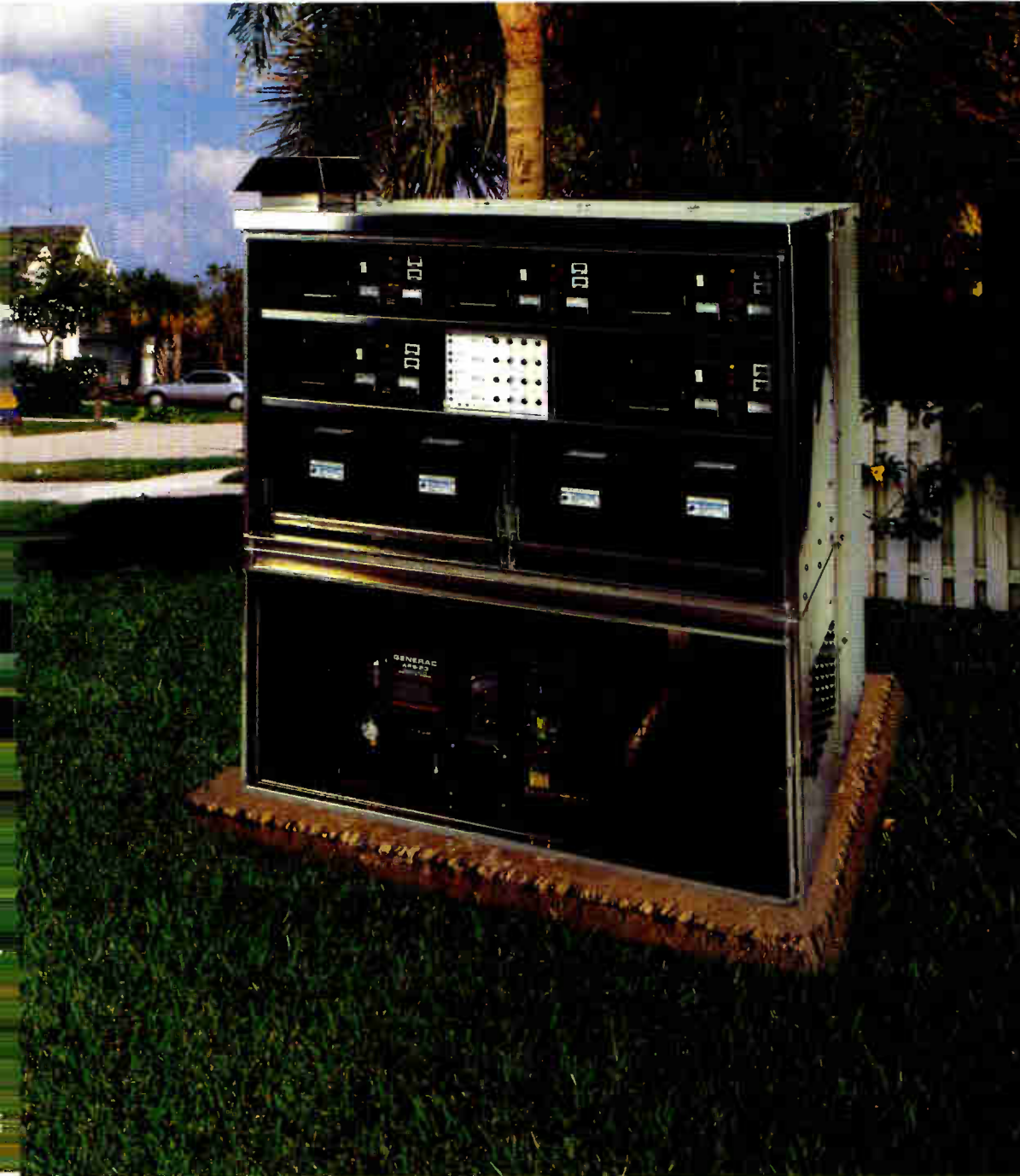
The doors have been removed for photographic purposes.
