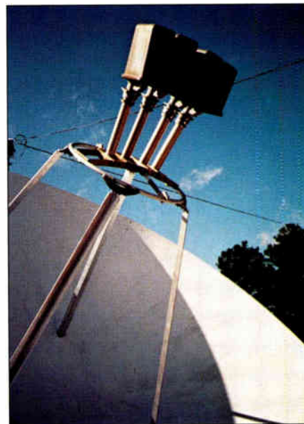
Multi-sat system on 5-meter dish.
