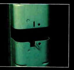
Knock out is easily removed with hammer and ordinary screwdriver.
