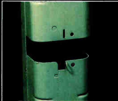
Knock out is easily removed with hammer and ordinary screwdriver.
