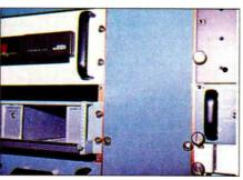
A 7-inch wide copper strip is installed from rack to rack
