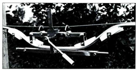
The use of mechanical cable shaping devices and cable placement rollers has greatly facilitated cable construction.
