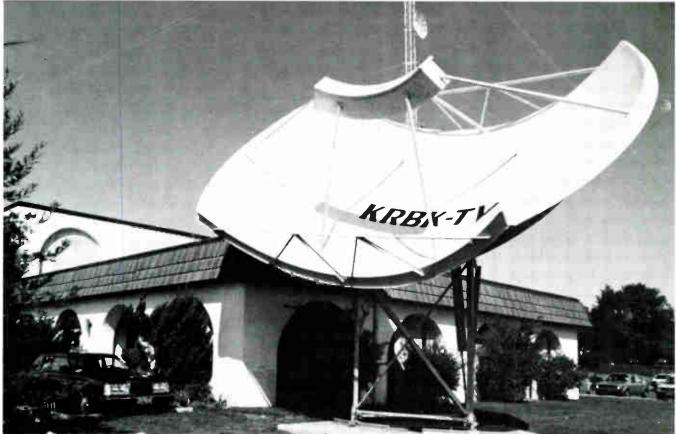
Only SIMULSAT<sup>®</sup> can see all domestic satellites at once with consistant performance on each bird. This means that you can see from Satcom I (135° W) to Comstar D3 (87° W) with the performance characteristics of a 4.6 meter antenna. This is the only existing antenna in the world to accomplish this.
