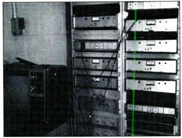
Zenith 14-inch color television supplying IF input to Scientific-Atlanta 6150 processor (note missing input converter).
