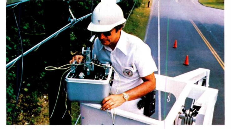
A Times field engineer splices a fiber optic cable, during installation, with a portable fusion splicer. Times supervises every installation to assure technical integrity and practical performance.
