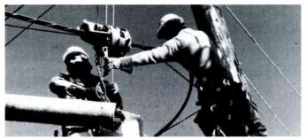
Installation engineers lash the fiberoptic cable onto the messenger wire in London, Ontario.
