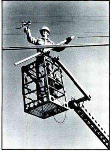
A member of Cablecom-General's construction crew strings a four-fiber optical cable from telephone pole to telephone pole in Joplin. The 3.56-mile aerial, fiberoptic cable replaces a conventional coaxial cable that carries video signals from the origination studio of Cablecom of Joplin/Webb City to the broadcasting tower on West 13th Street in Joplin. The smaller, lighter fiberoptic cable (attached to the pole held by the crewman) is easier to handle than the heavier coaxial cable seen below.
