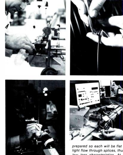
It was check and double-check in Valtec's stringent preparations before shipping the fiberoptics/cable communications system materials to Las Vegas. At top left, cable is colorcoded so that each fiber can be identified to allow installers to choose the proper sets. At top right, fibers at cable end are
