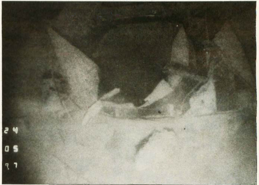
Photo 3: The gaping hole left by the collapse of the Titanic's first (forward) smokestack. The huge liner had four smokestacks.
