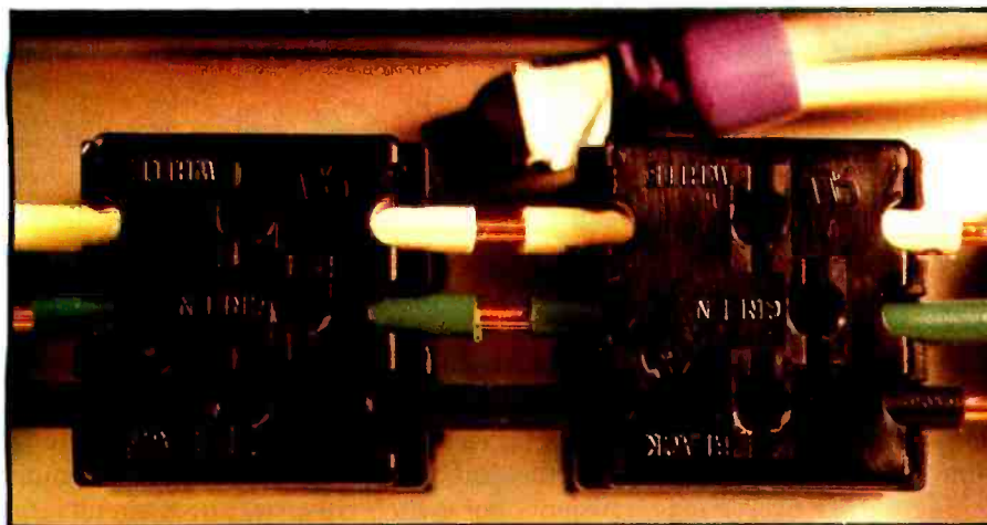
Photo 4: Using an X-acto knife or similar tool, strip insulation from the wires between the receptacles (which I number 1 through 4, from left to right) according to the following system: between 1 and 2, strip the green and black; between 2 and 3, strip the green and white; between 3 and 4, strip the black and white.
