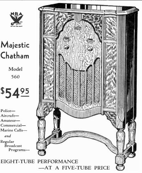
This five-tube radio uses three of the new Majestic "Duo-Valve" tubes, thus making it actually an eight-tube set in performance, as these three tubes each do the work of two ordinary tubes.
