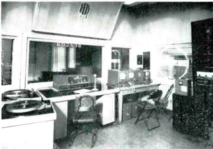
COMPLETE CONTROL ROOM AT R.E.T.S. FOR AM, FM, OR TV.
