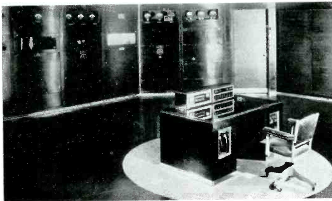
WOR Transmitter and Control Desk
