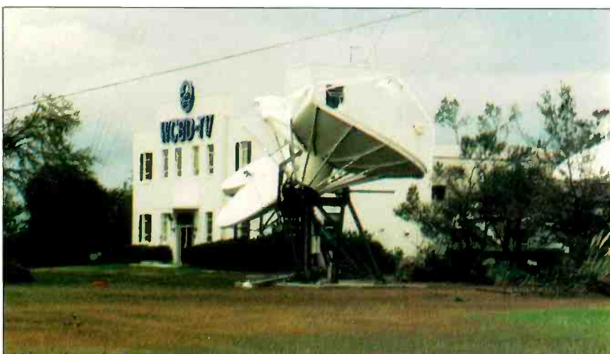
WCBD-TV's satellite dishes were bent out of shape by the storm.
