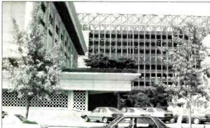
The International Broadcasting Center in Seoul, under construction adjacent to KBS headquarters.
