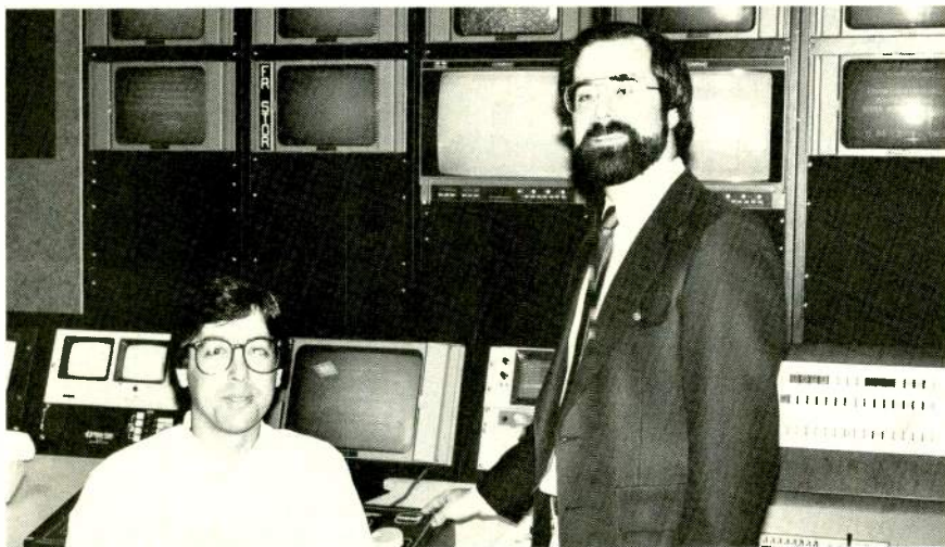
Richard Mandeborg, technical coordinator, computer graphics, left, and Lenard Pearlman, VP, technical services, in one of the facility's 3/4-inch rooms.
