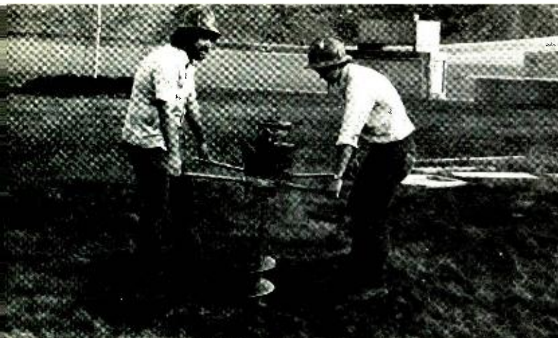
Stages in antenna installation. Hand-held drill prepares the holes
