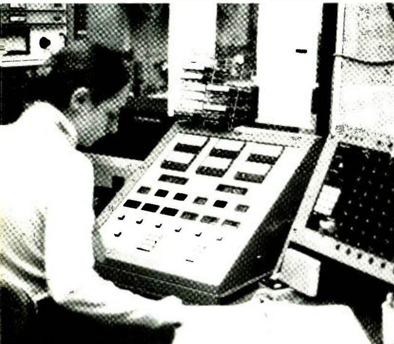
Election-night newscasts on the CBS Radio net will be distributed to various sections of the net at this control position in New York. Operator selects portion of net to receive broadcast by simply pushing a button on panel. Emergency "net alert" panel is on the right
