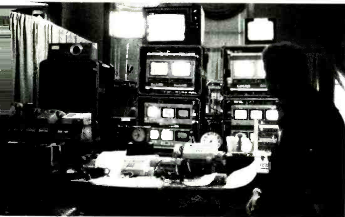
The overall mobile switching center stacks up and goes into operation within five hours
