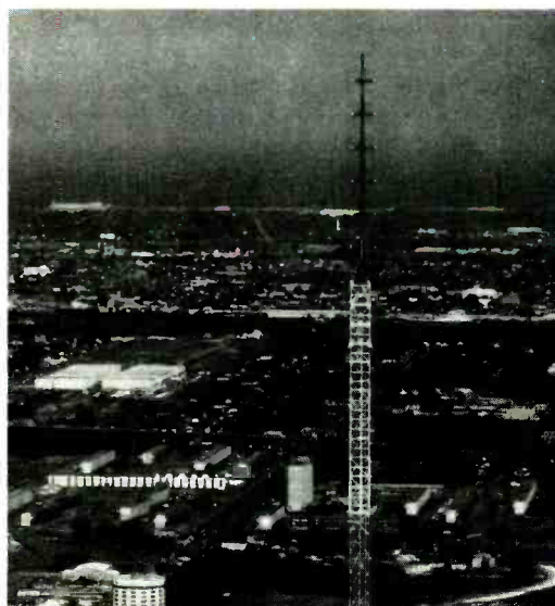
WWL-TV, New Orleans, Louisiana, CPV omnidirectional antenna. No tower change required.
