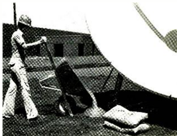
Holes are filled in with concrete for stability
