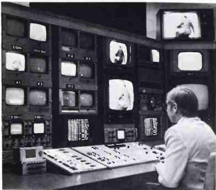
Through the use of automated switching, master control operators have been reduced from five to three people: master control console operator, a film chain operator, and a VTR operator. Master Control man has plenty of time to keep a sharp eye on monitors.
