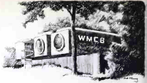
Through use of pre-fab modules, WMCB was able to use sloping terrain and preserve trees.
