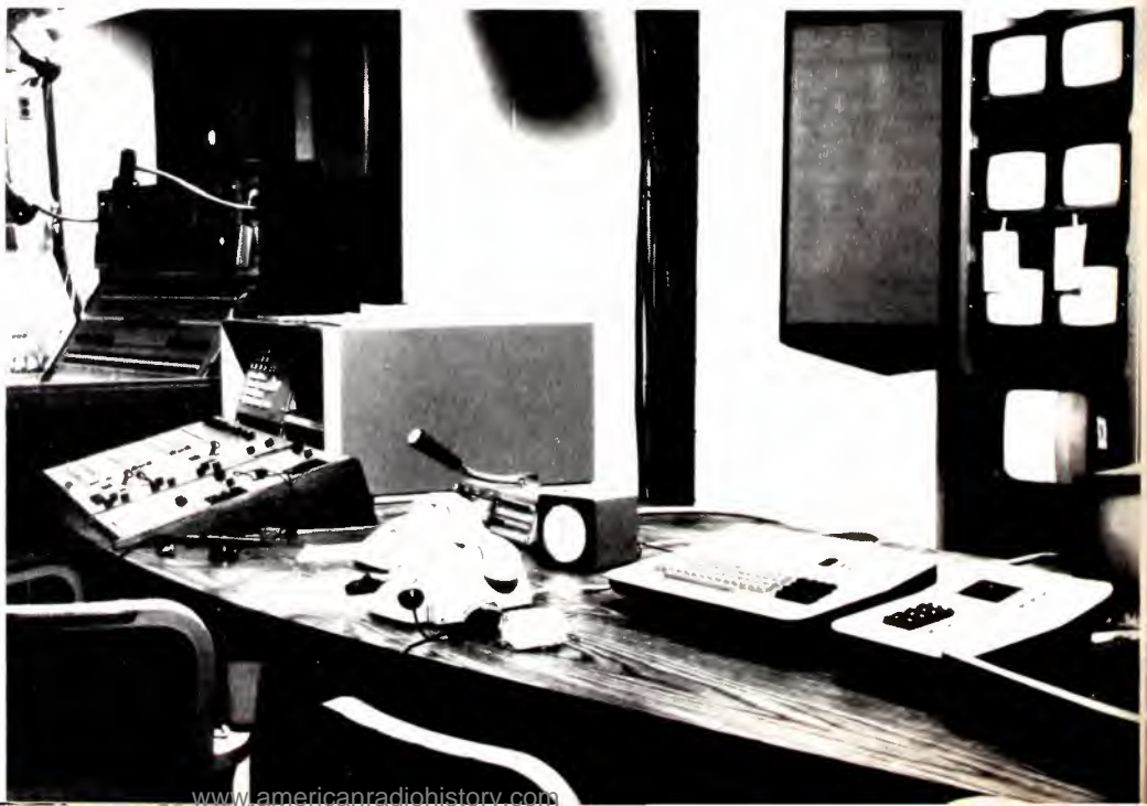
General view of Studio A audio-video control room. Audio console is to the right. Through the window is the lighting control room.
