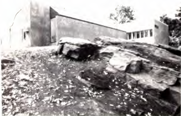
Rocky site added to construction effort, but variations in level were turned to advantage by architect, to give building a commanding position
