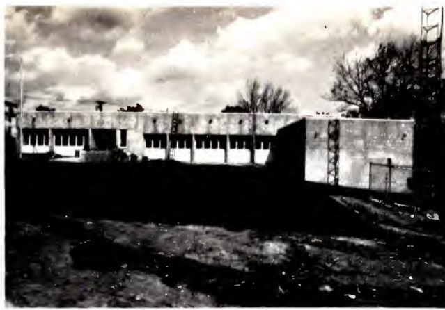
Exterior of building during construction with, at right, housing for mobile news crew, and main entrance left of center in facade.
