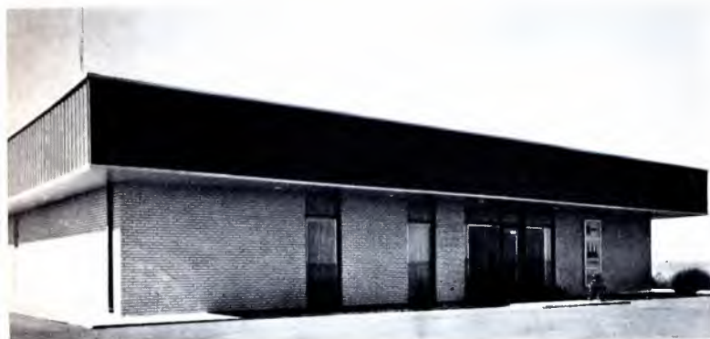
The home of KWKA-FM and KTOM-FM is a 3600 sq. ft. building made up of components produced by Stran-Steel Corp., a Subsidiary of National Steel Corp.
