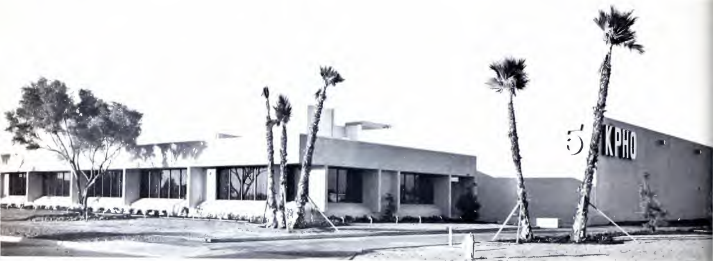
KPHU located away from downtown and could go single story on a 3½ acre site. Total floor space in the new plant is about 43,000 sq. ft., compared to approximately 20,000 in the old building. There is room for an anticipated computer installation.
