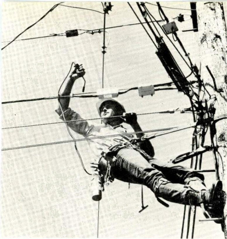
Utility poles are common denominator for power, telephone and CATV systems.
