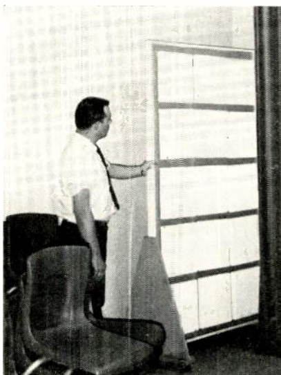
Absorbent panels on wheels used in studios at WGBH-FM in Cambridge, Mass., can be moved to best location for room tuning.
