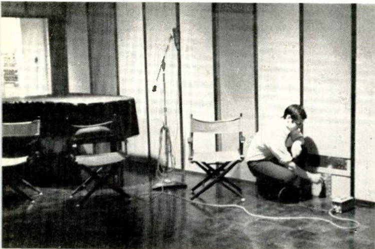
Alternating absorbent and reflecting wall panels "tune" Petrucci & Atwell recording studio in Boston.
