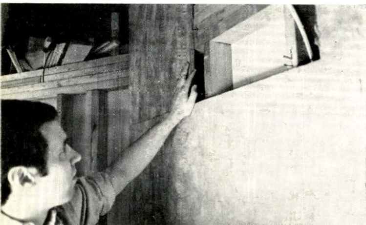
Bob Petrucci points out room-within-a-room construction used in his studio. Double layers of sound-absorbing material help isolate room from street noises.
