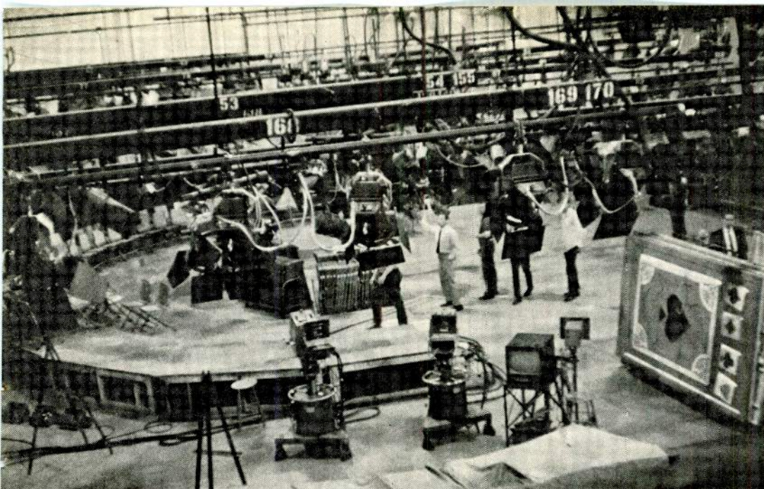
Technicians keep busy in Studio 5, giving it many faces in a broadcast day. Here, they adjust positions of quartz lights on their overhead pipe battens.
