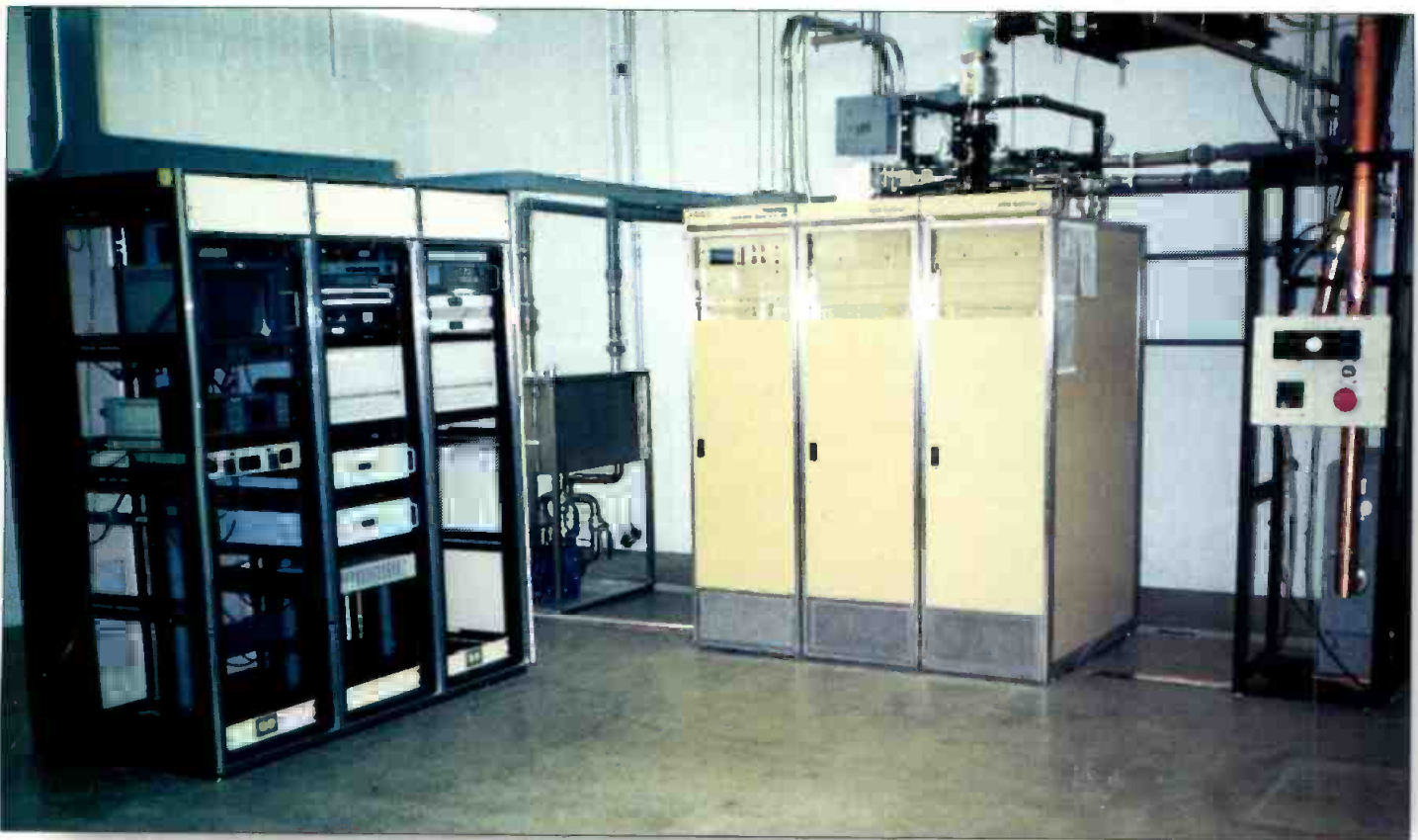
Station WLWT-DT, Cincinnati, OH, selected an Itelco T603WN, solid state, liquid-cooled transmitter for its channel 35 DTV needs.
