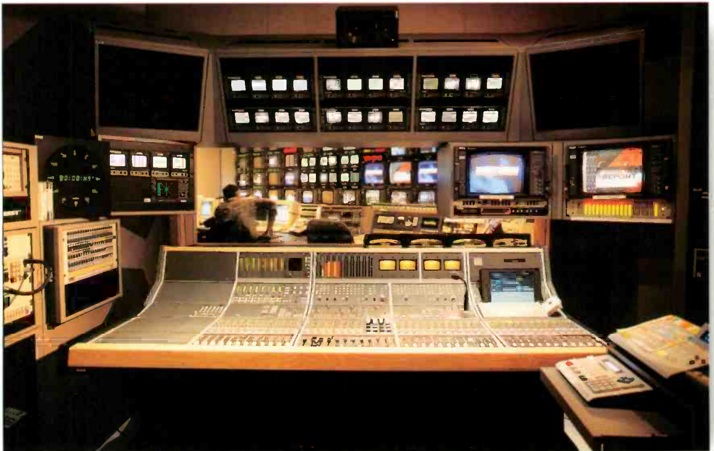
Production Control Room 9 uses digital monitors with programmable under-monitor displays to support 10 operating positions.
