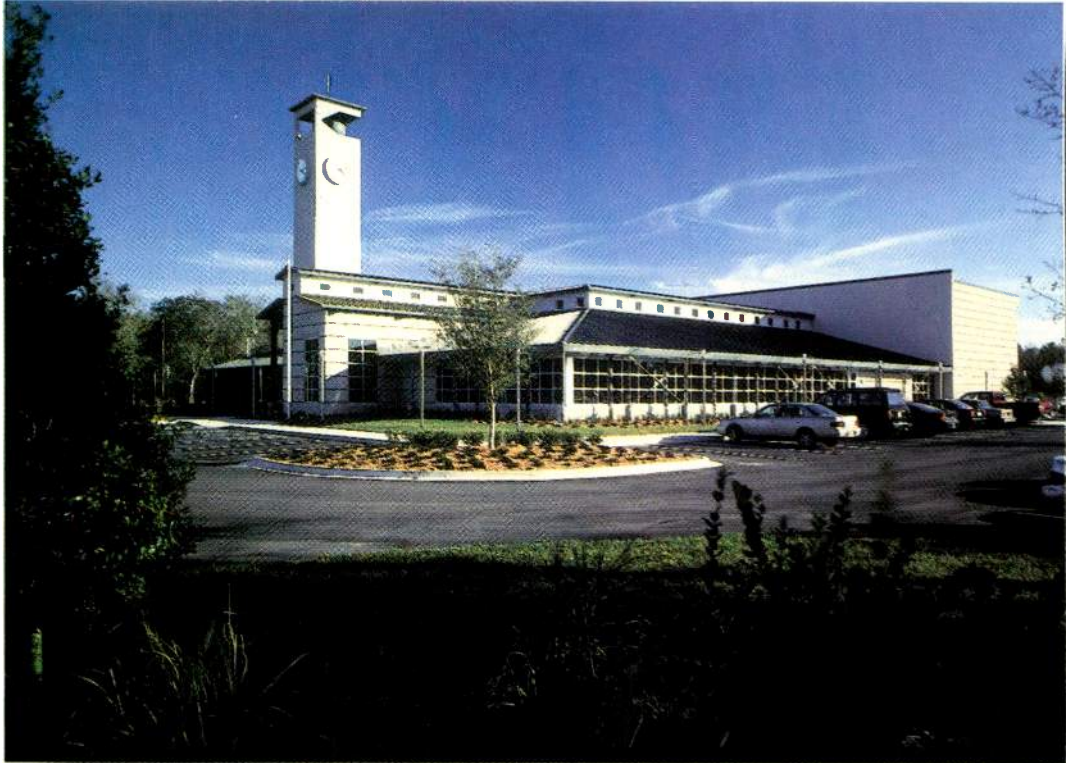
View of front of building exterior/main entrance, northeast view.
