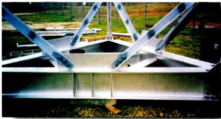
New tower top cap to be installed. A four-inch steel plate will support a 32,000-pound antenna system. (Photo courtesy of Jay Watkins.)
