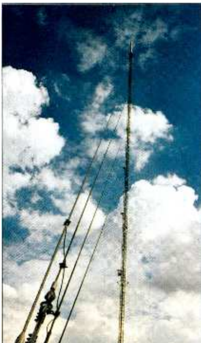
This 1,767-foot LeBlanc tower located in Homestead, FL, is believed to be the heaviest tower in the world. It is designed to withstand hurricane-force winds and replaced a tower that collapsed during Hurricane Andrew.
