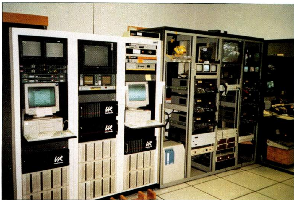
At KIMO-TV, Anchorage, AK, three separate streams of automated programming are recorded and played back using a combination of tape and disk-based storage.
