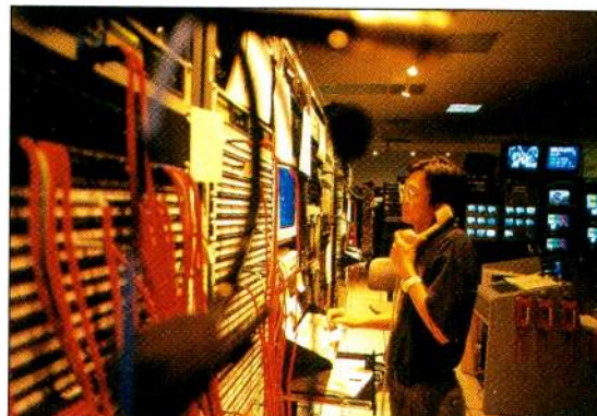
Willie Yau sets up the CSEDIT editing software for controlling and assigning of the Telex RTS 400x400 ADAM digital matrix intercom system at NBC's BOC.
