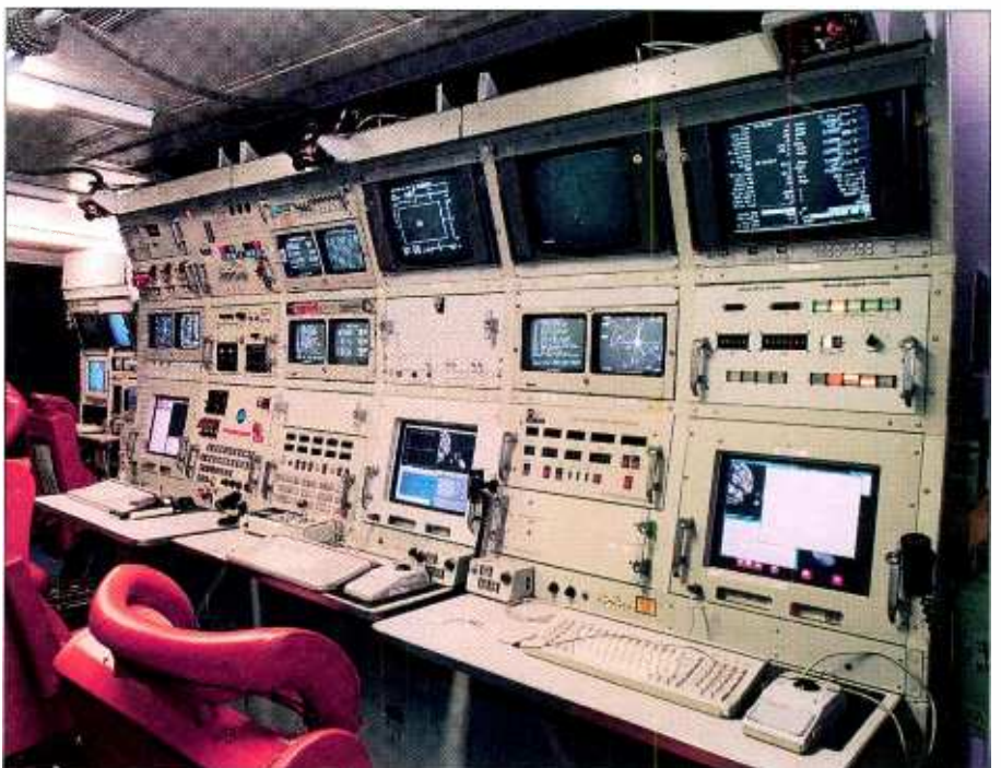
The mission director console occupies the middle of the cabin area. Researchers occupy the area toward the front (left of picture), and the ACTS/BAT and audio/video equipment and personnel were stationed aft.
