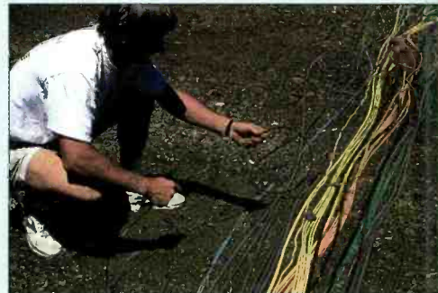
During NBC Sports' broadcast of the Celebrity Golf Classic in Lake Tahoe, NV, a technician examines a single fiber-optic cable that is transporting the same signals carried by all the other (copper) cables alongside it. (Courtesy of Lightwave Systems.)
