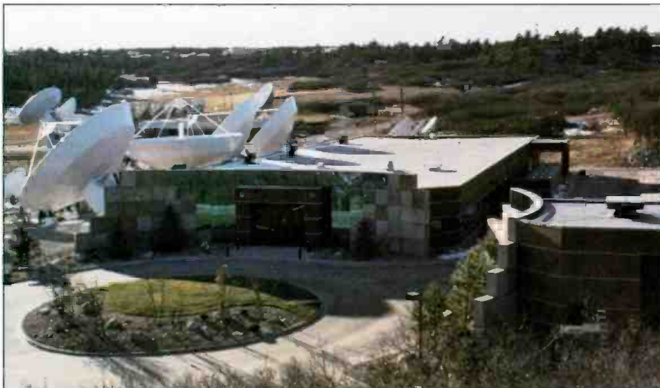
DirecTv uplink facility in Castle Rock, CO, showing surrounding protective terrain. Four large dishes at left carry main uplink transmissions; the other smaller dishes at center rear receive incoming feeds. The building in the right foreground houses emergency generators. The building at left rear and its surrounding dishes are the control center for the Hughes fleet of communications satellites.
