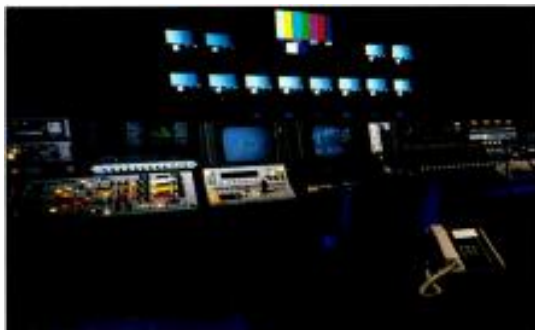
DIGITAL FINISHING ROOM
