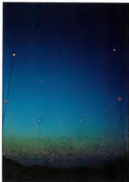
The 12-tower array of Dallas' KLIF-AM.
