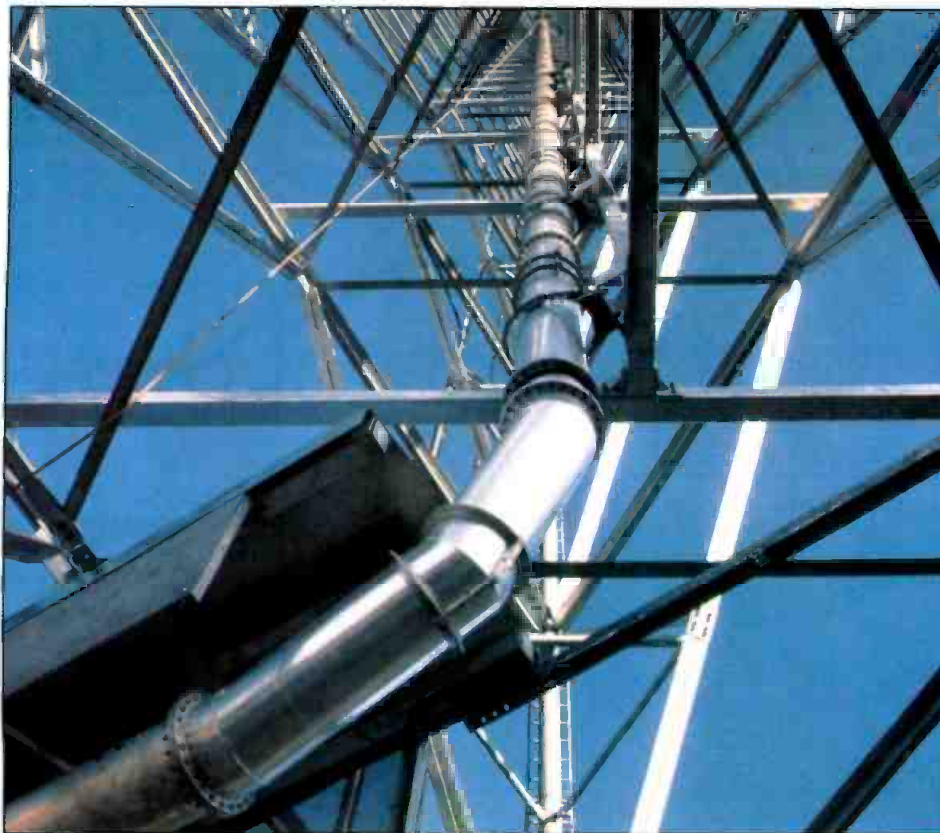
The 90° circular bend made it possible to use circular waveguide from the transmitter to the antenna.
