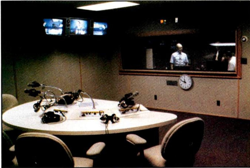
Some studios are equipped with three TV monitors, allowing an announcer to translate a live event while viewing three different network feeds.
