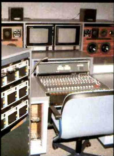
The technical director console under construction in the control room of Studio 4. Video monitors can be seen in the background. A total of 28 black-and-white continuity monitors are used, plus three color monitors (program, preset and preview).
