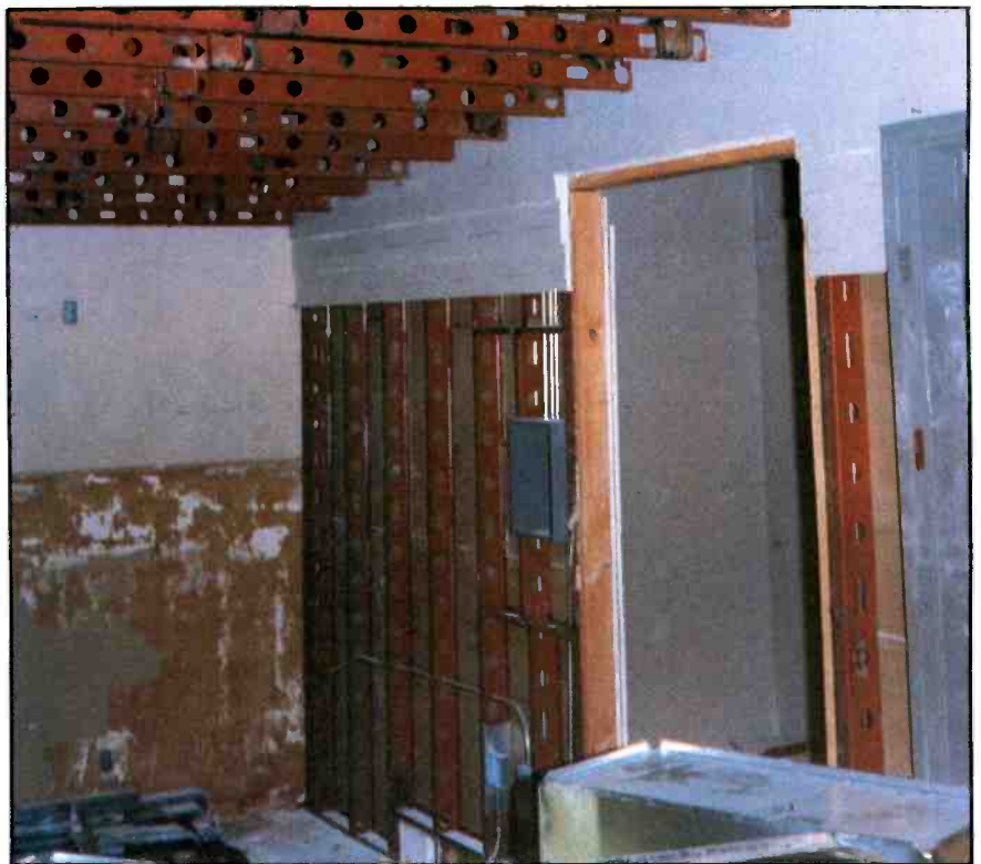
The Studio 4 audio mixing room under construction. Note the sloping ceiling and three layers of overlapping drywall. The studs are 14-gauge steel.
