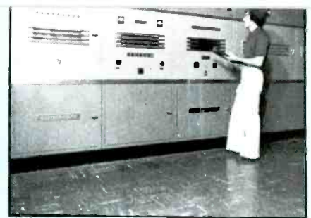
A WWSW-AM staff member reads the individually metered parameters on the Westinghouse transmitter-of-license.
