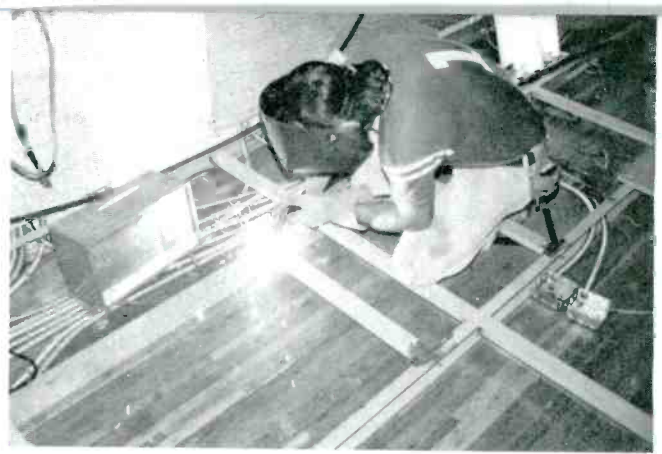
The subfloor is rewelded for added strength.
