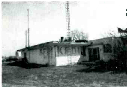
Original KFDI Facility
